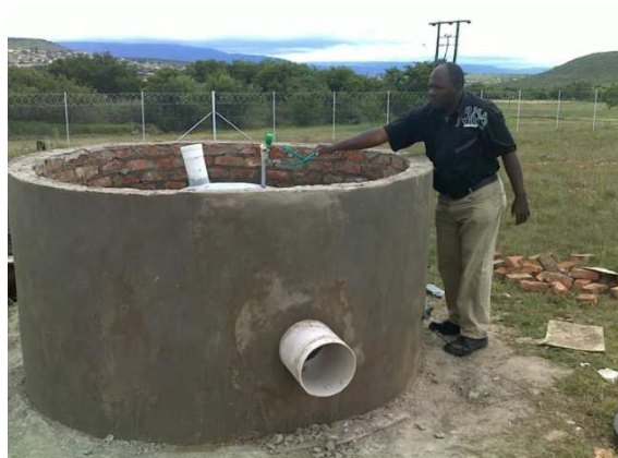
Figure 4. The Plastered second wall digester.
