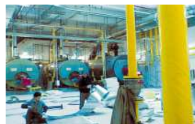
Figure 1. Basement Boiler Room.
